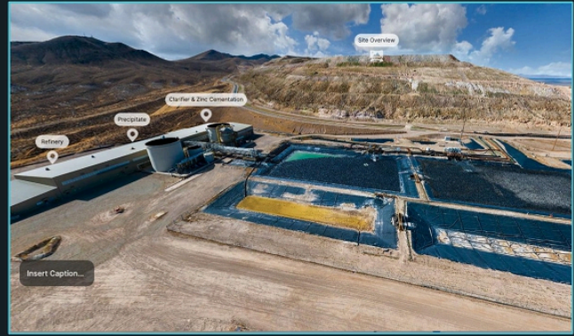
NORTH MERRILL-CROWE PROCESSING FACILITY
