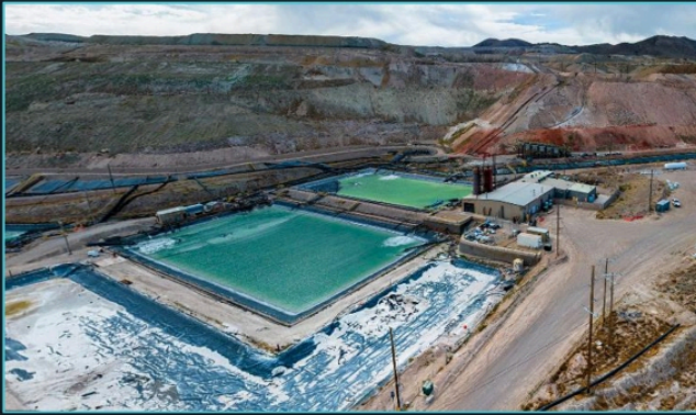
BRIMSTONE MERRILL-CROWE PROCESSING FACILITY
