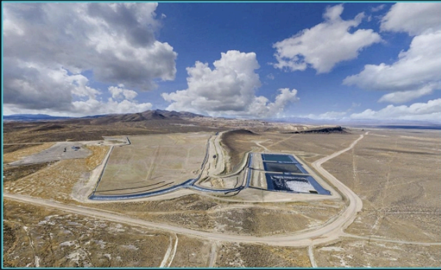
NEW LEACH PAD - PERMITTED AND AVAILABLE FOR ORE LOADING
